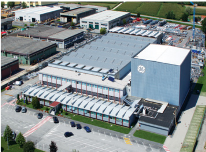
Competence Center for Disconnectors in Noventa di Piave, Italy
