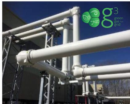
420 kV GIL - SF 6 -free with g 3 gas mixture
