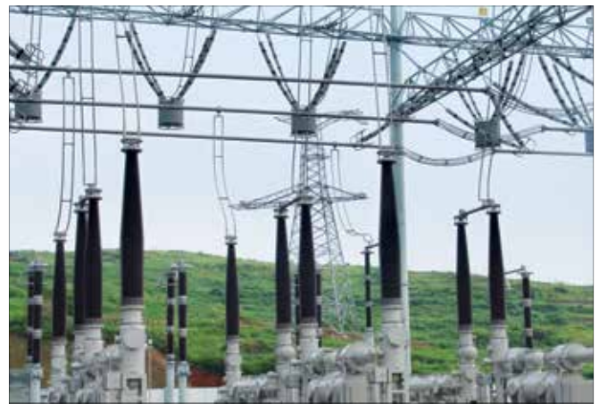
550kV Hybrid Gas Insulated Switchgear
