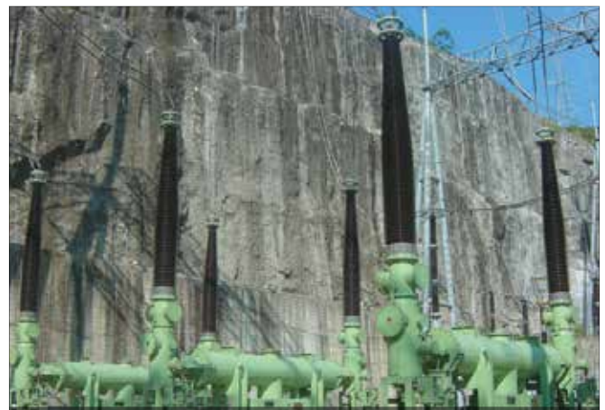
550kV Hybrid Gas Insulated Switchgear
