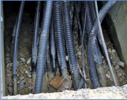
Extensive amounts of copper cables need to be distributed from each switchyard apparatus back to the control house
