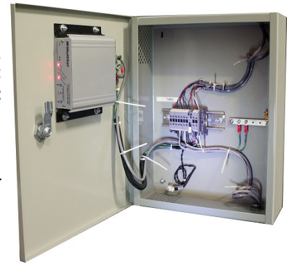
Battery junction box (BJ BATT)
