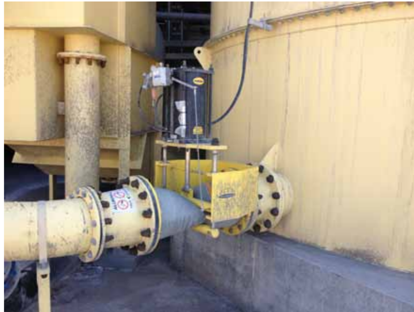
Tank level control valve - smooth flow deflection
