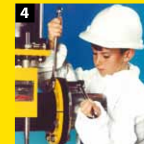
4 Replace backing flanges and flange bolts
