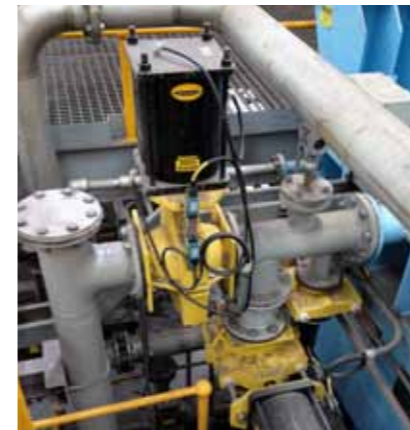
Various Enclosed Pneumatic Pinch Valves with limit switches
