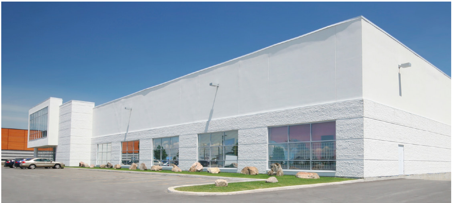
Commercial building with 200A nominal service, 277V.
