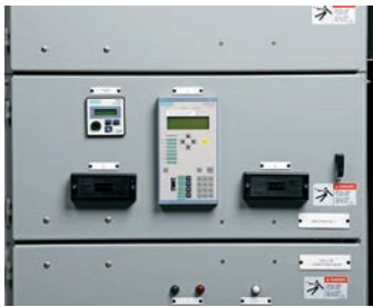
Figure 10: Central compartment for panel devices
