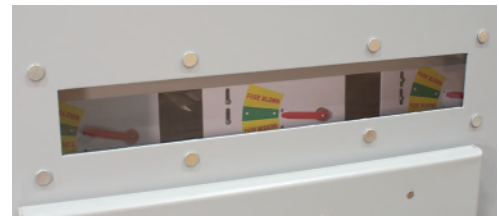
Blown fuse window with indication flag
