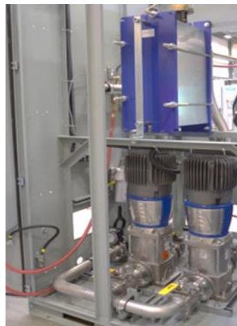
Example of integral liquid-liquid heat exchanger
