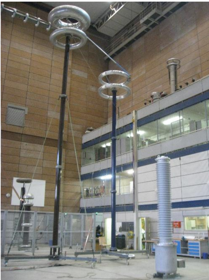
STEF 420 during routine test
